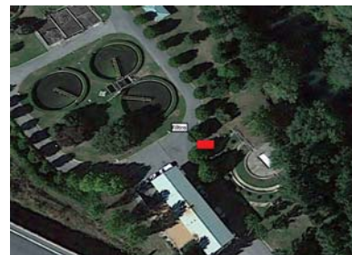
WWTP of Estella
