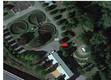
WWTP of Estella
