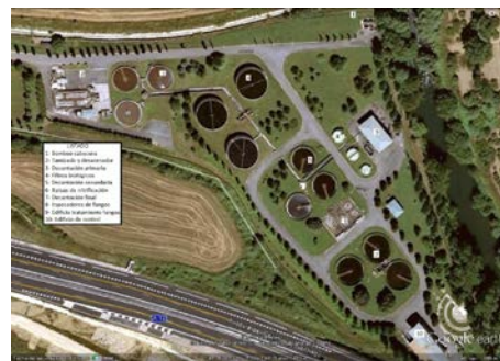
WWTP of Estella
